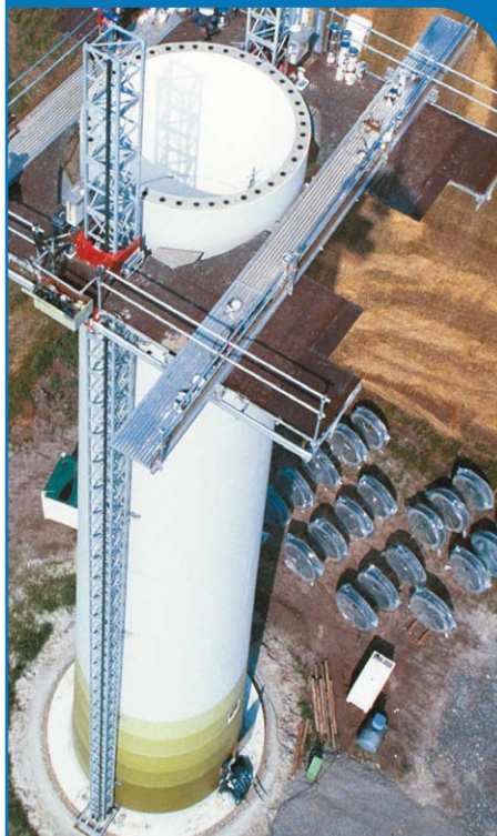
Prestressing ducts and tendons (on ground) for precast concrete onshore wind tower. Images courtesy of the Concrete Society
