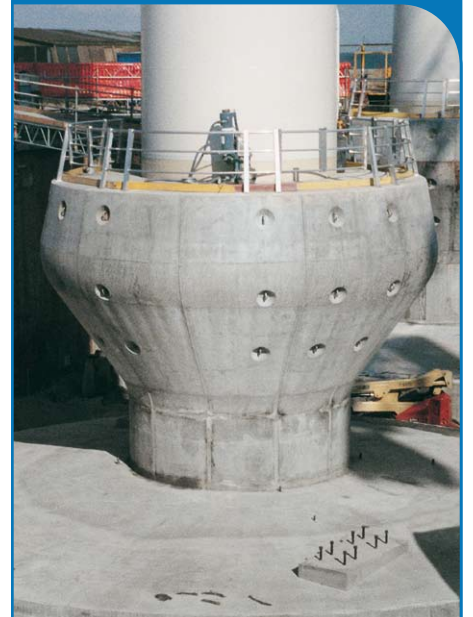
Concrete gravity foundations enabled onshore prefabrication of pylon sections.
