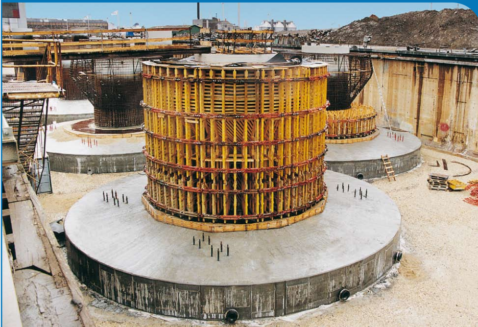
Complicated foundation profiles possible using innovative, circular formwork solution.
