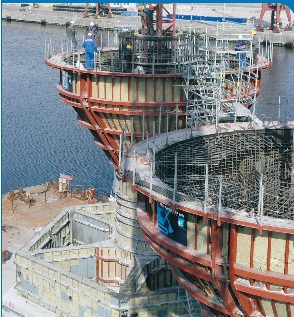
Onshore construction of concrete gravity foundations for 9km offshore wind farm development, Denmark. Image courtesy of The Concrete Society
