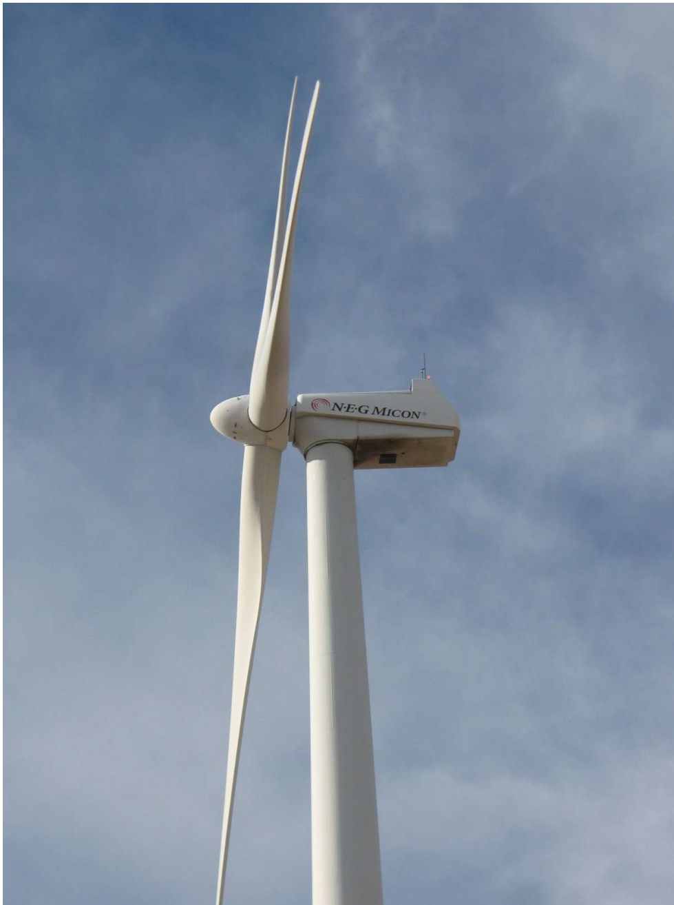
Figure 1.1 — A vintage wind turbine up close. The turbine is the visible part of a wind farm, but everything that supports it — from foundation to grid connection — is the Balance of Plant.
