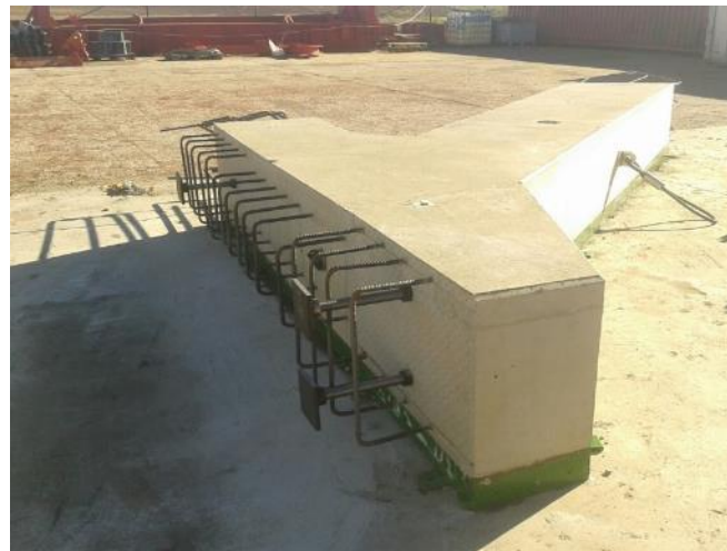
Braces for diverse windfarms, some precasted on-site, some precasted in precast plant facilities (but open air – upper left case)
