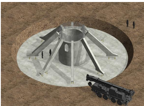
5 Braces installation
