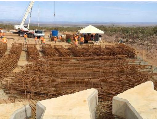
Braces for diverse windfarms, some precasted on-site, some precasted in precast plant facilities (but open air – upper left case)
