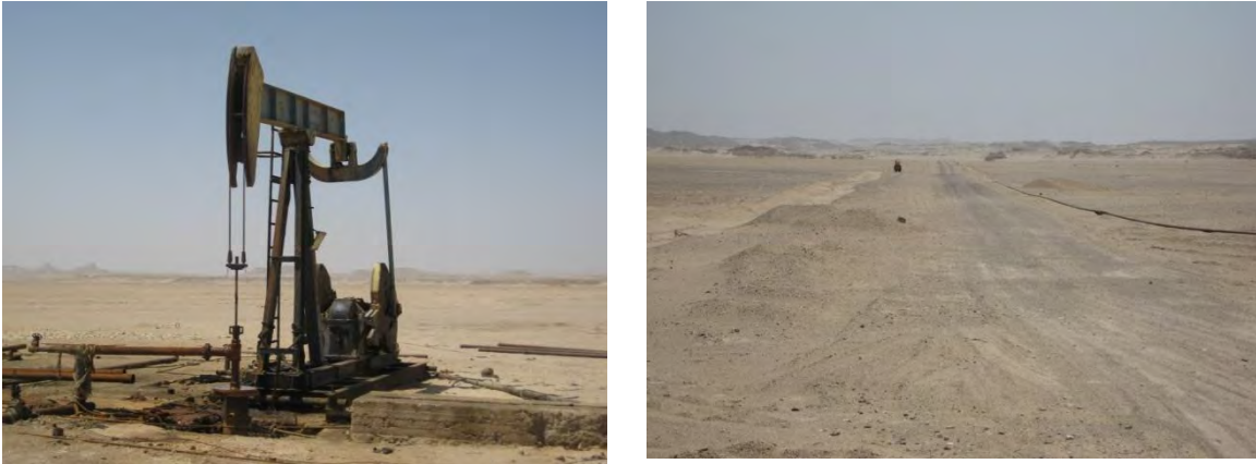
Fig. 4.5: Water pumping, water pipeline, buried MV cable and access road
