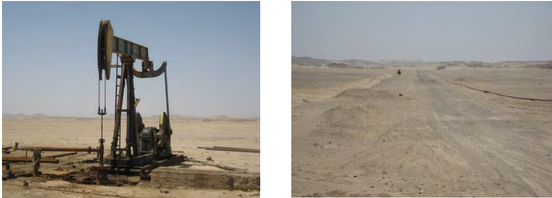
Fig. 1.6: Water pumping, water pipeline, buried MV cable and access road
