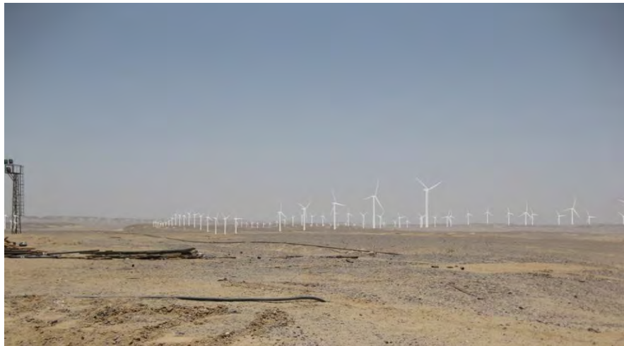
Fig. 5.1: Visualisation from GPC temporary office facilities about 1 km in the East of the Project area
