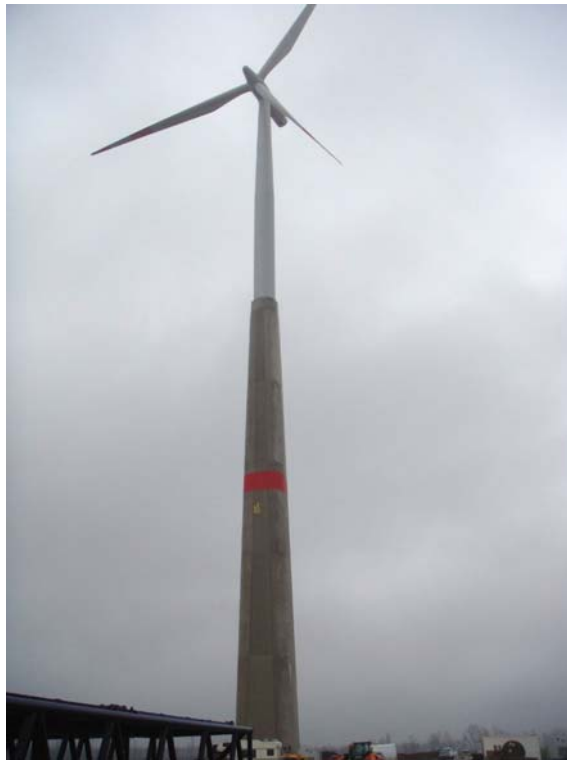
Figure 7 – Hybrid concrete and tubular steel tower.
