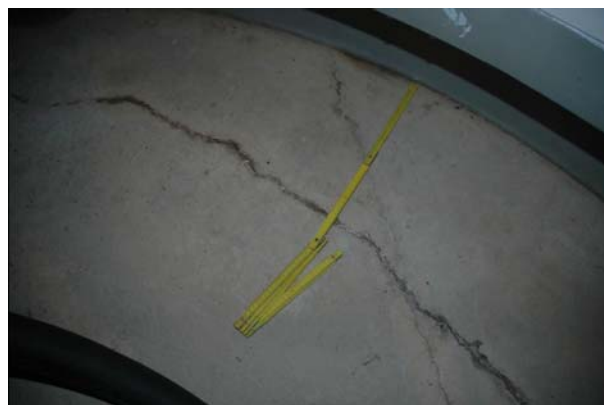
Figure 39 – Significant crack approximately 35 cm from the tower, [15].
