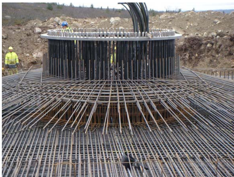
Figure 21 – Flange on the top of the pedestal before casting.
