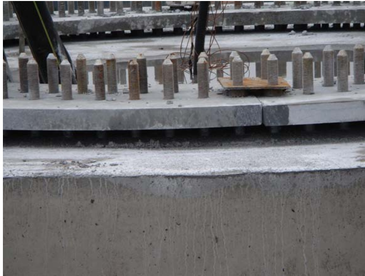
Figure 22 – Flange on the top of the pedestal after casting.
