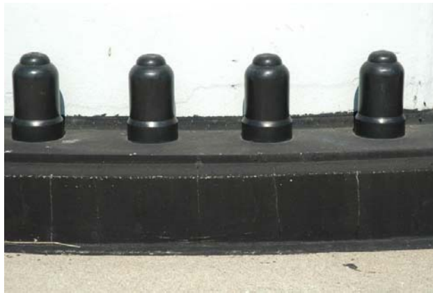
Figure 28 - Vertical shrinkage cracks, [15].
