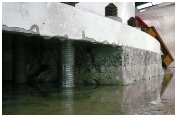
Figure 32 – Two different mortar grouts are used, [9].
