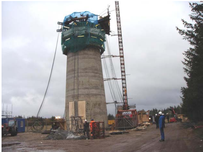
Figure 6 – Production of prestressed cast-in-place and slipform cast concrete.
