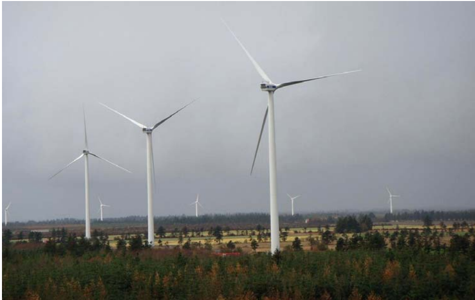
Figure 5 – Towers made of prestressed cast-in-place and slipform cast concrete.
