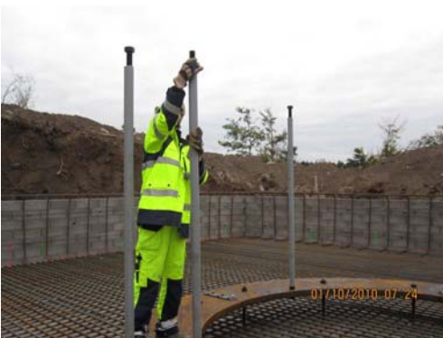
5- Stud bolts and bottom ring
