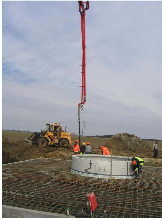
Figure 24 – Pouring of concrete in a prepared spread footing formwork, [13].
