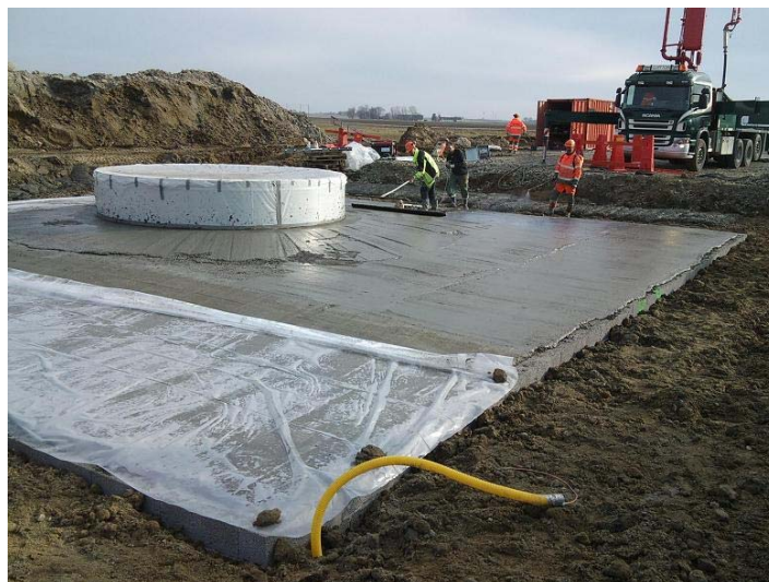
Figure 25 – Trowelling of the surface and covering the surface by plastic foil to prevent drying during curing, [13].
