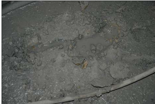
Figure 40 - Spalling (s) due to the cracks, with out-flowing water, [15].
