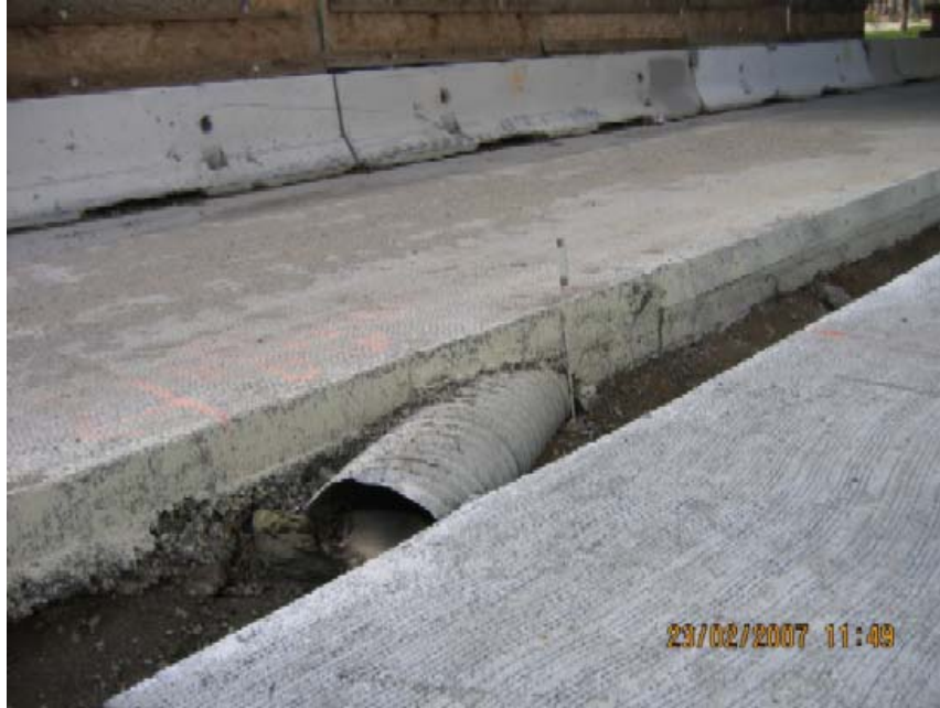
Figure 12 Drainage Crossing Constructed without Cover
