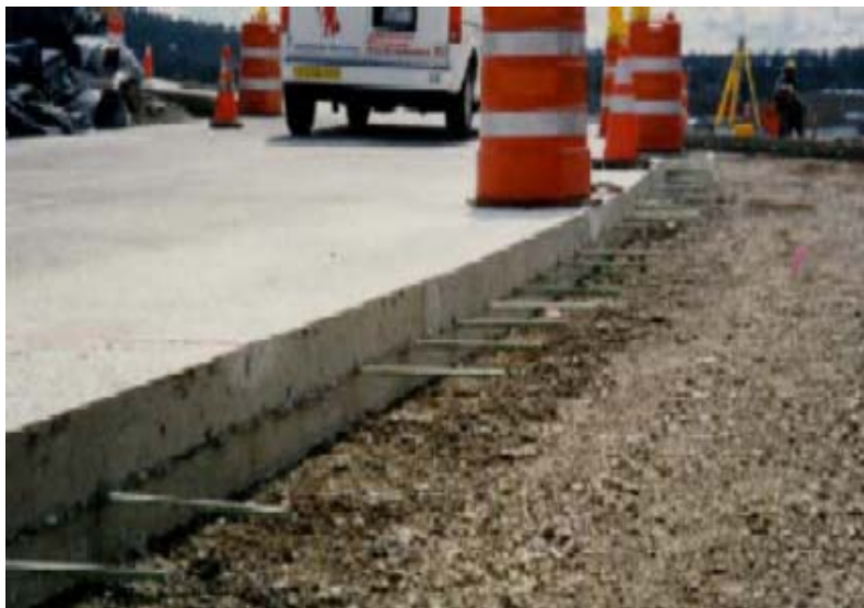
Figure 4. Tie Bars in a Longitudinal Joint
