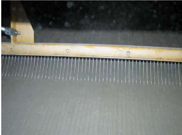
Figure 20. Steel Tine Device Being Used on Concrete Pavement
