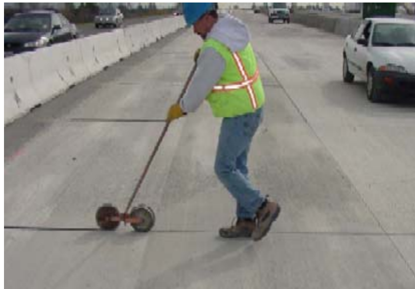
Figure 18. Backer Rod being Pressed Down with Steel Roller
