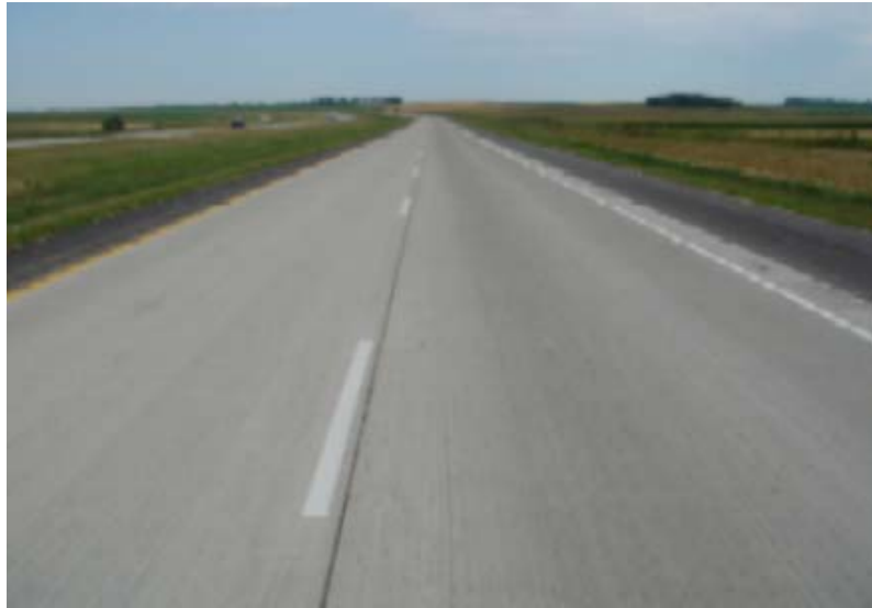
Figure 3. Longitudinal Joint at Lane Line
