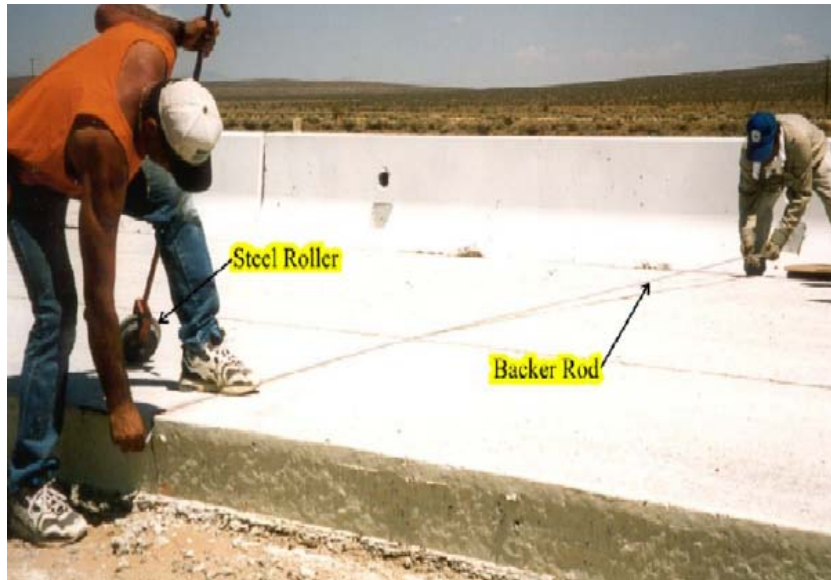
Figure 17. Backer Rod being Installed
