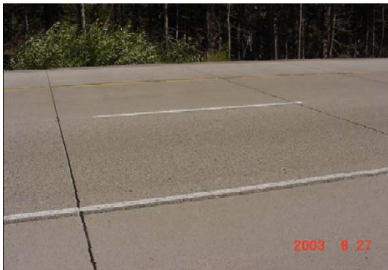
Figure 2. Transverse Joints Perpendicular to Lane Lines and Longitudinal Joints
