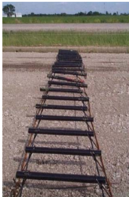
Figure 13. Misaligned Dowel Bar
