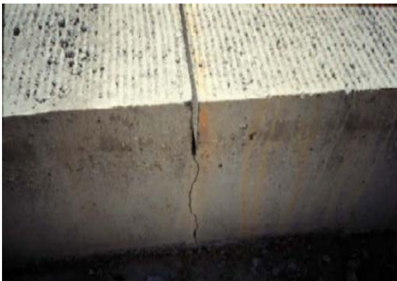
Figure 9. Aggregate Interlock Across Transverse Joint
