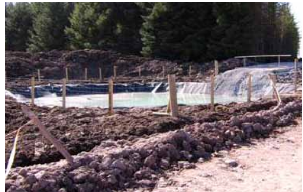
A well designed and located cement wash out bay can prevent bad practice elsewhere on site. A ticketing system to ensure it is used by all drivers has been shown to be useful.
