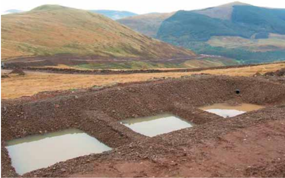
In some locations substantial constructed 'Step' designed settlement lagoons maybe be required to manage large volumes of contaminated run-off.
