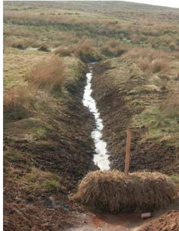
Straw bale 'pinned' in place.
