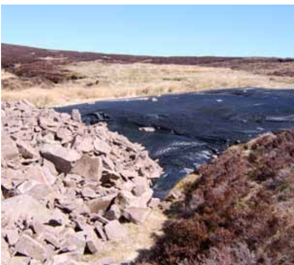
Poor floating road construction e.g. attention to detail is required at track edges to prevent construction material spilling onto surrounding vegetation. Please refer to the Floating roads on Peat guidance.
