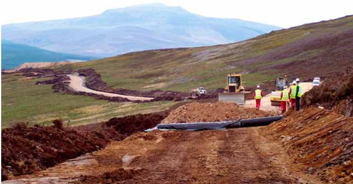
Construction of a cut road.
