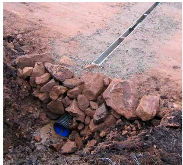
Culvert under road – better attention to detail would 'hide' the exposed pipe.
