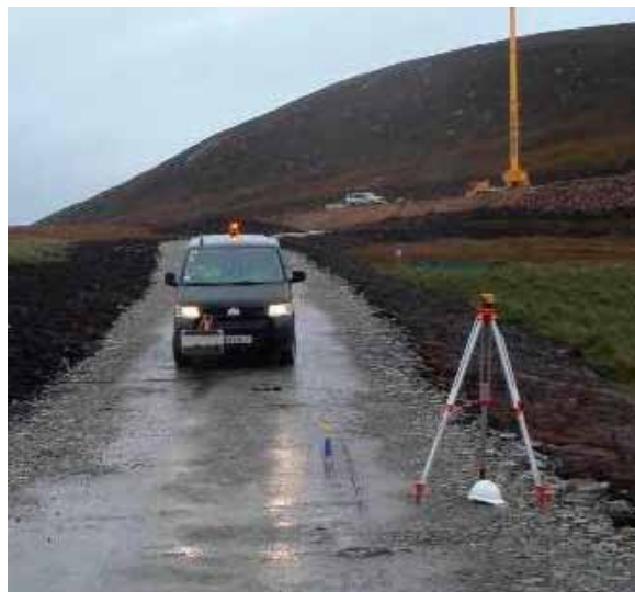
Surveying floating road structural integrity. Note that excessive material should not be placed on the side tracks as shown on the left of this image.
