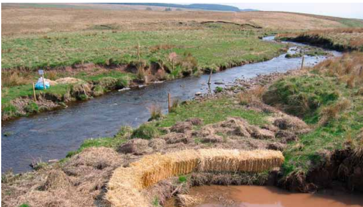
Sediment lagoons should always be situated away from watercourses, unless, as in this case, there are no alternatives. Better pre-construction planning should address this.
