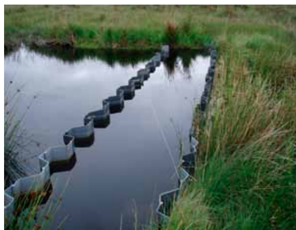
Blocked drainage ditch using plastic sheet dam.
