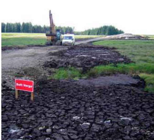
An example of bad practice. Excavated peat placed 4m from edge of access track. Note that no peat turves have been re-used. This peat is likely to dry out and provides no ecological benefit.
