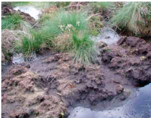
Peat dam blocking water flow in old forestry drainage ditch. The peat may slump and in time the dam becomes ineffective. In addition, to improve stability, peat turves should cover the top.
