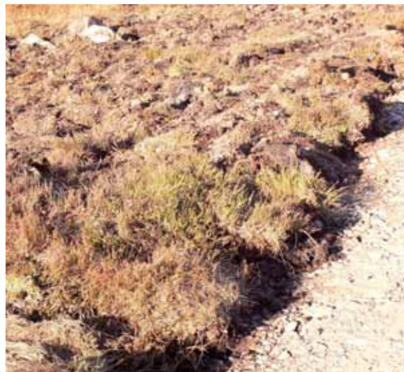
An example of good practice. Reinstated turves at road verge provide optimal restoration. Careful supervision of works may be required to achieve this.
