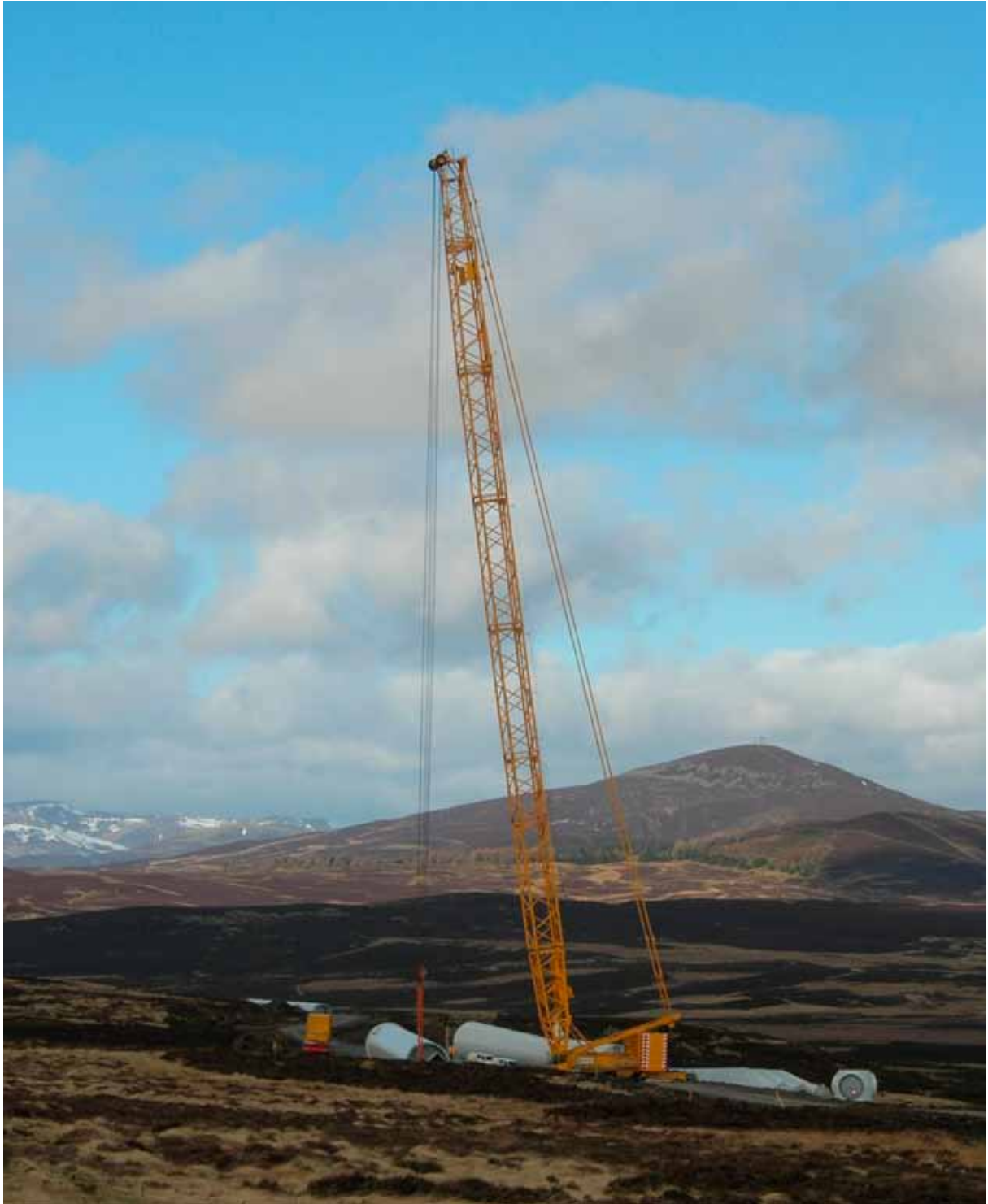
Careful micro-siting of crane pads will be required to minimise longer term impacts.
