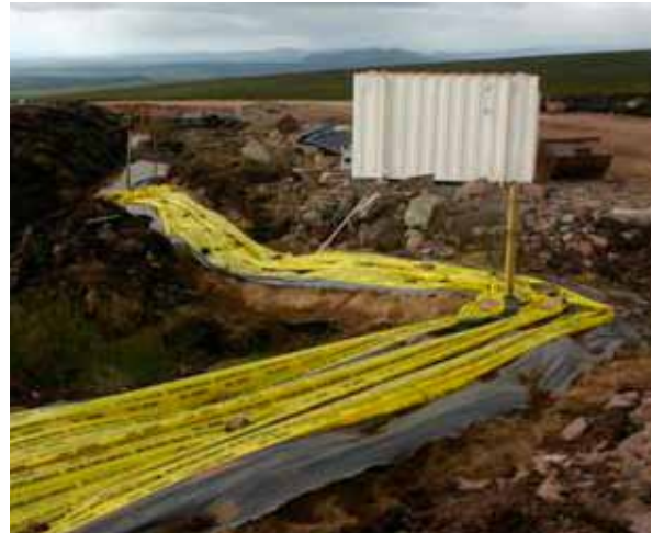
Cable trench adjacent to constructed road.
