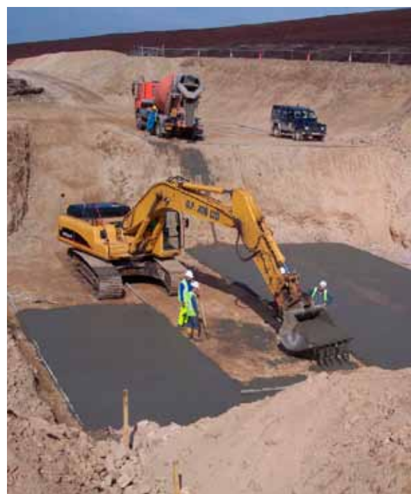
Preparation of turbine foundations.
