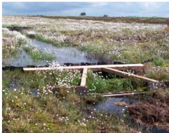
Good practice: Blocked drainage ditch (plastic sheet dam in centre of photo) with Sphagnum sp.
