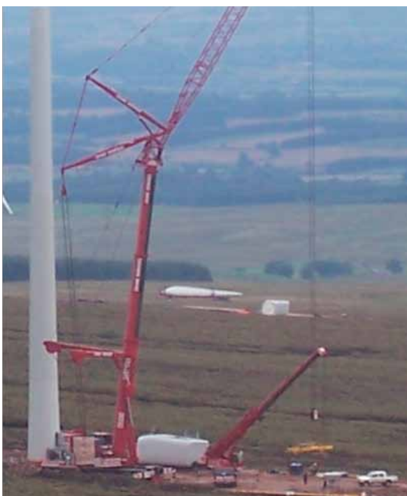
Lifting of final turbine components.
