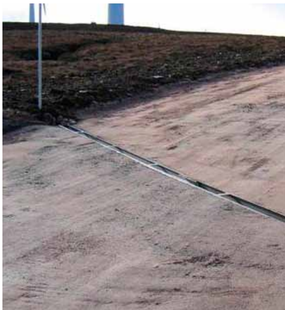
Cross-drain on access track.
