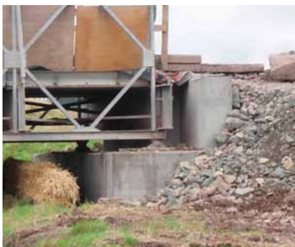
Bridge and bank habitat. Steep sides of loose material could be washed off in a storm event. Use of splash boards on bridges can prevent contamination of watercourses and is an example of good practice.
